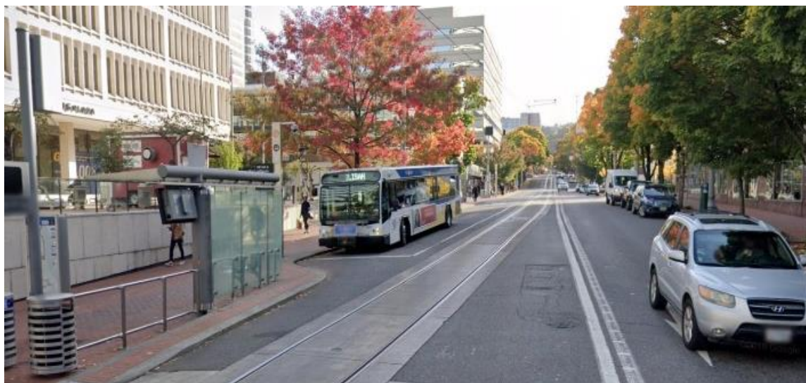
Figure 9 Mall qualities: Bus stop, bus bay, and sightlines of light rail (Google Earth)
